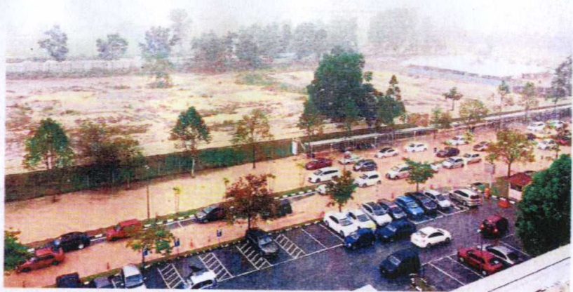
Worrying: The Sultan Abdul Halim Hospital parking lot was flooded during the downpour in Sungai Petani.
